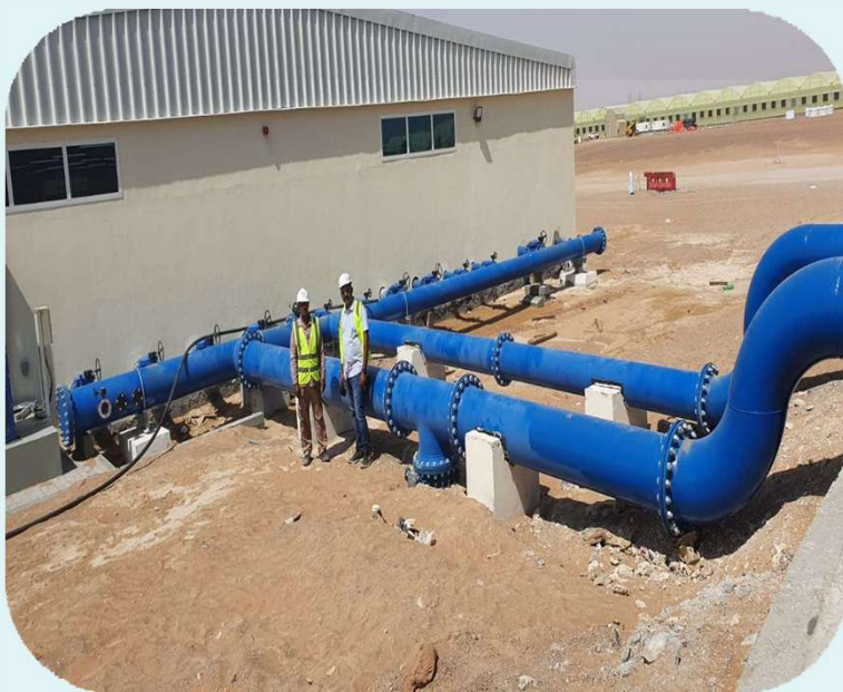
Main contractor: DUTCO TENNANT LLC Project: AL Foah farm development Scope of work: Pipe Fabrication and Installation
